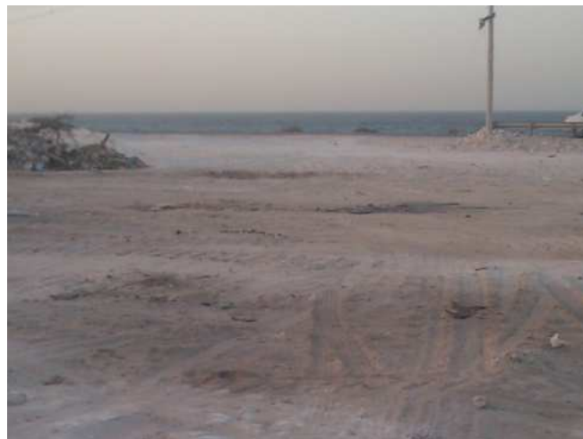
Figure 7: Damping the Waste and Leveling the Earth Surface
